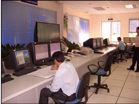
Operation of Phu My switchyard
