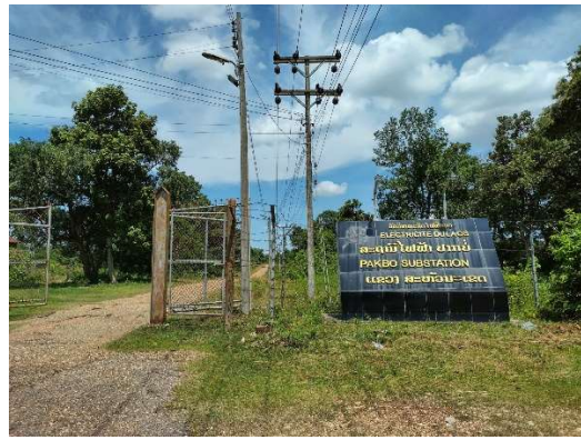
Pakbo Substation (Entrance to Substation Site)
