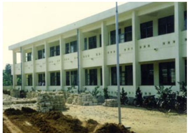
A primary school building provided by the project. The school playground is being developed through donations from the children's parents.
