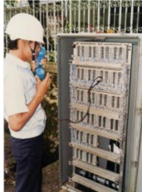
A counterpart carries out a telephone switchboard test.
