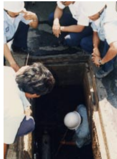
Counterparts inspect underground telephone lines.
