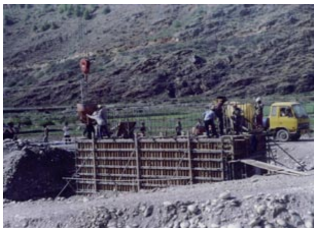
A bridge under construction
