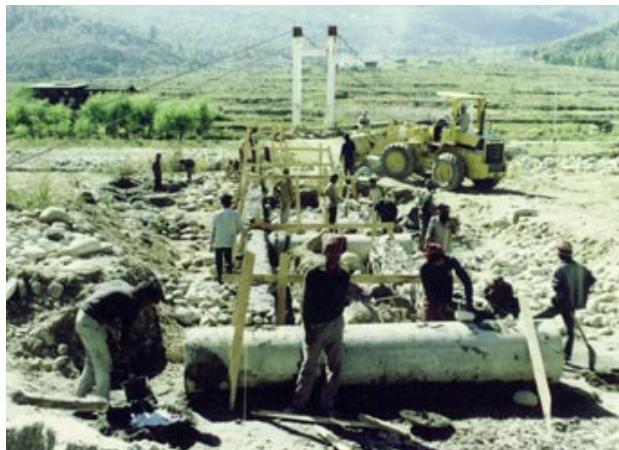
Provided equipment is being used to pave a connecting road to a bridge built with grant aid
