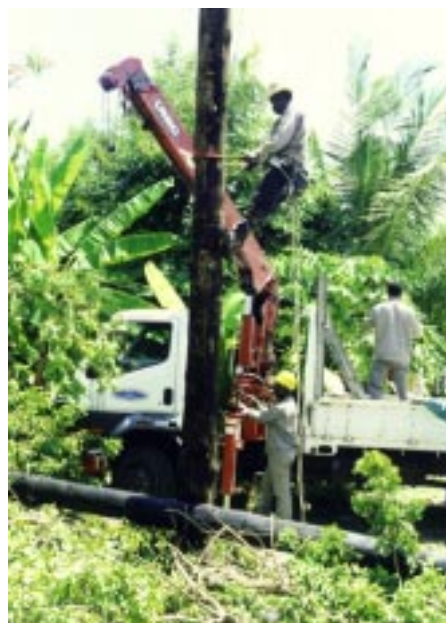
Counterparts changing an electric pole
