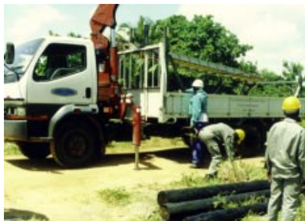
Counterparts carrying out maintenance activities
