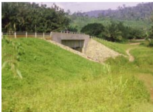
A bridge that has been constructed. Maintenance conditions are favorable.
