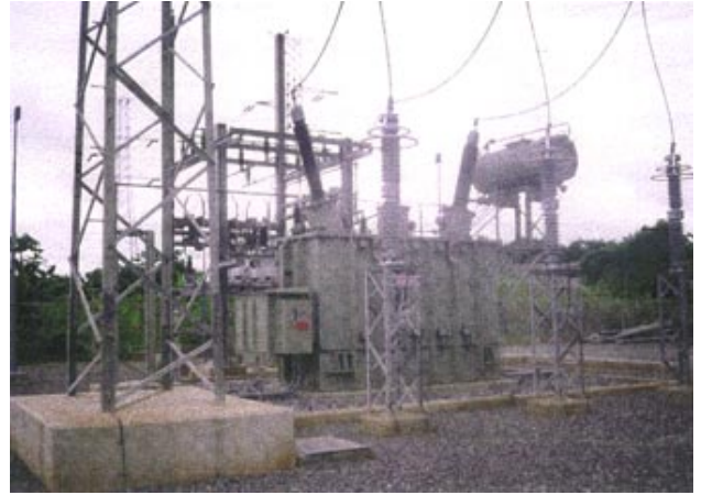
A newly installed transformer substation
