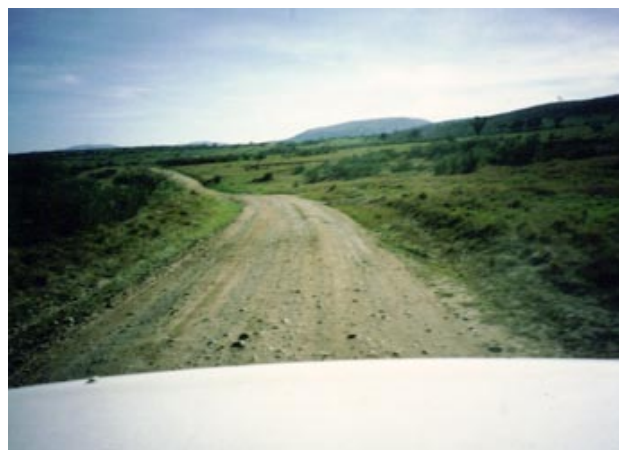
A graded road
