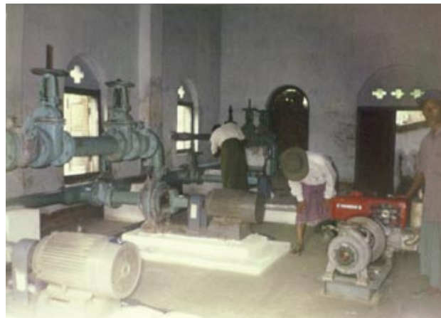
Booster pumps installed in a pump shed
