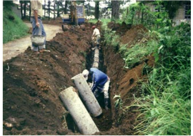
Sewage pipes continue to be laid in the city of Baguio
