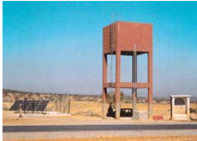
A water tank with a solar panel (Rural Water Supply Project in Morocco)
