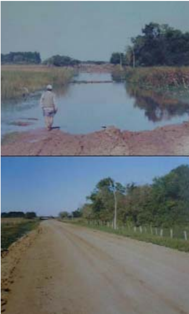
Upper: Flooded trunk road Lower: Same road improved by the Project (The Rural Development Project in the Region South of Pilar in the Paraguay)
