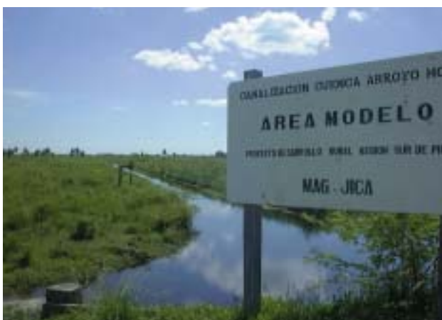
Drain load constructed by the project
