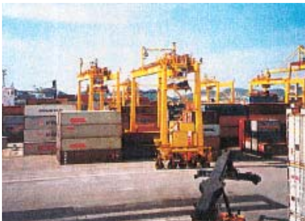
Thailand / Development Project of Leam Chabang Coastal Area
