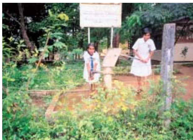
A well constructed by the project
