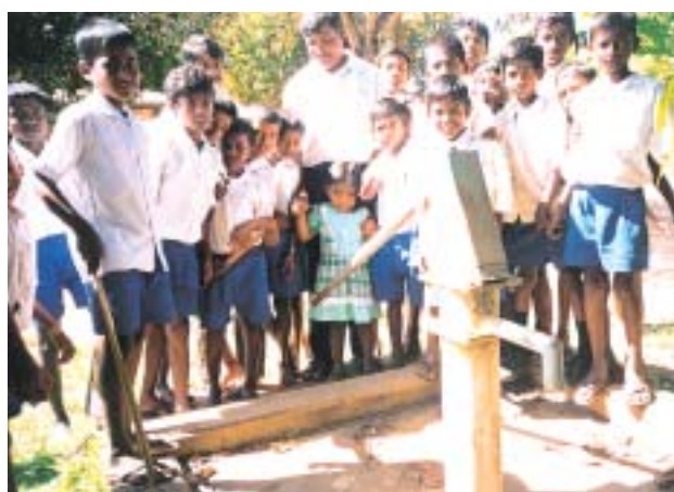
A well constructed at an elementary school
