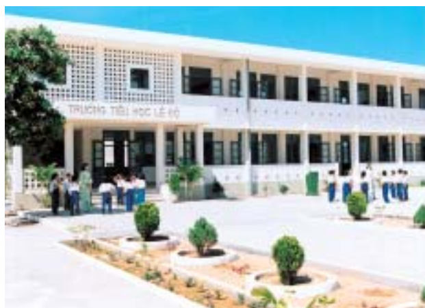
Elementary school constructed by the Project
