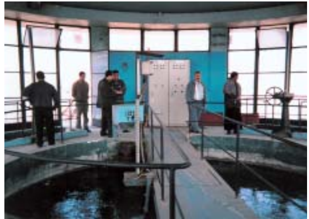
Water treatment facility
