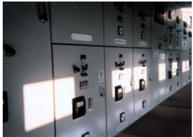
Electric operation board
