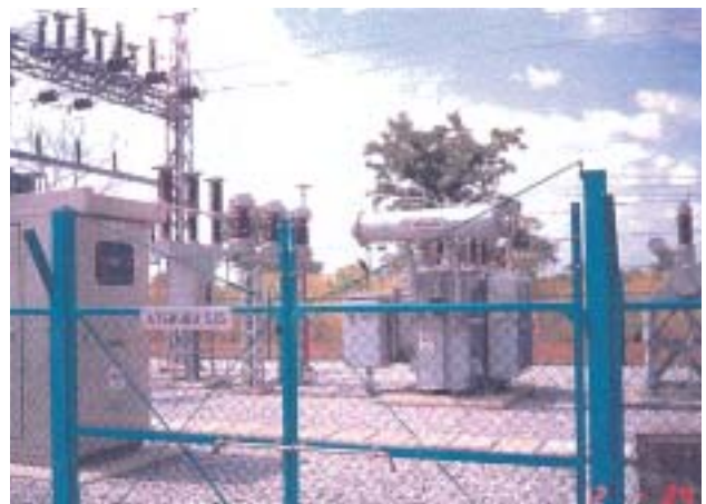
Booster Station at Atebubu area
