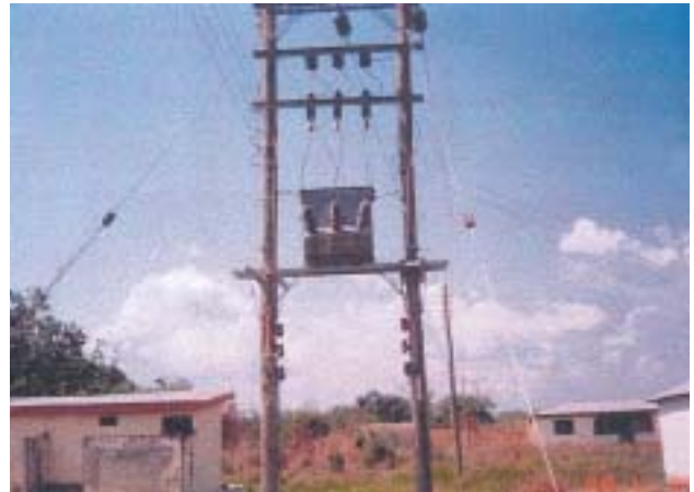
A transformer placed on a telegraph pole
