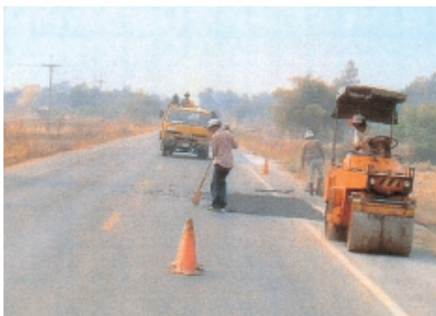
Maintenance of Route 199 'Project for Bridge Construction in Northeast Thailand'
