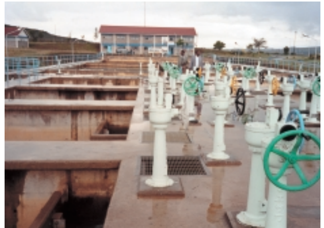
Water purification plant under Greater Nakuru District Water Supply Plan (constructed by Yen-loan)
