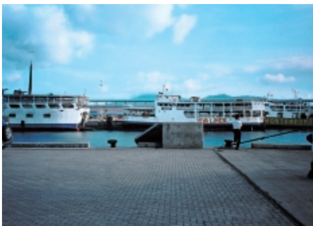
The Batangas Port (Passenger ship terminal)
