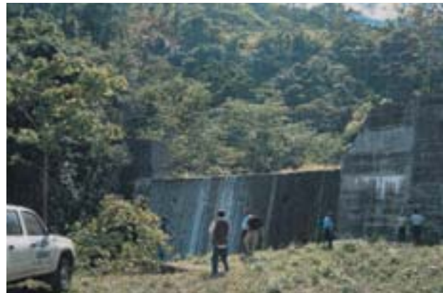
Mudslide-control dam by the “Project for Flood Control along the Choloma River”.
