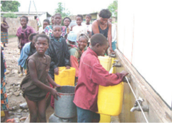
Public water taps in the George Compound (The Program for Improvement of Living Conditions in Zambia)
