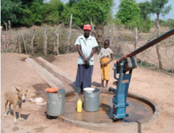
A borehole water supply system using a hand pump, which was constructed under the project (Project for Rural Water Supply in Binga District in Zimbabwe)
