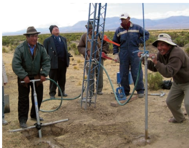
People digging a well by hand drilling
