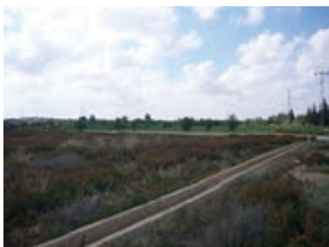
A concrete farm ditch
