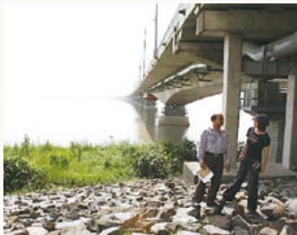
Jamuna Multipurpose Bridge which has power line and gas pipeline attached to the road
