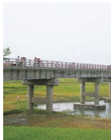
Bridge constructed by the project (Jamalpur District)
