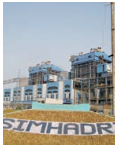
Simhadri Thermal Power Plant
