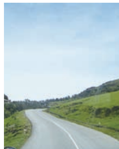
Rehabilitated Dili-Cassa Road
