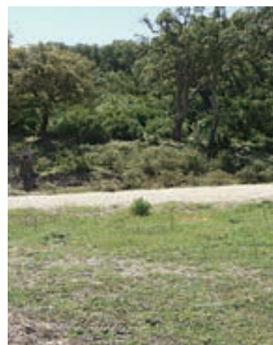
Forest road constructed by the project
