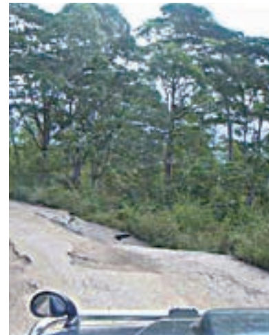
A road with surface damage
