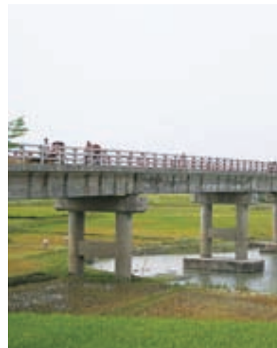
Bridge constructed by the project (Jamalpur District)
