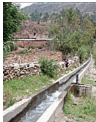
Irrigation channel constructed by this project
