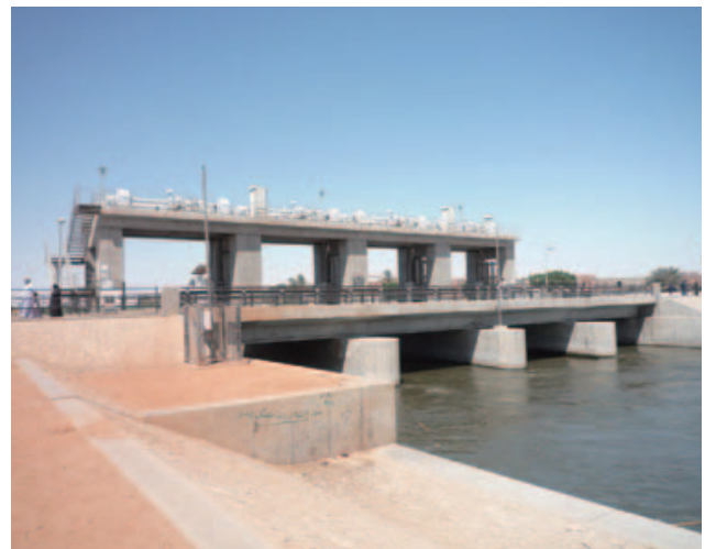
A rehabilitated and improved Sakoula Regulator (Egypt)
