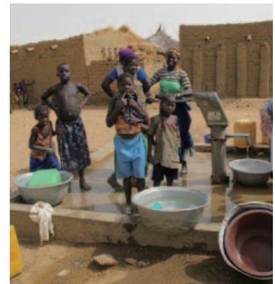
A borehole with a hand pump provided by the project
