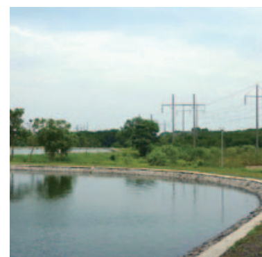
Stabilization pond at the wastewater treatment plant
