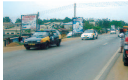
The road rehabilitated by the Highway Sector Investment Project. Heaviest traffic between Kumasi and Cape Coast.
