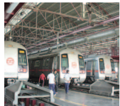
Train shed in Shastri Park
