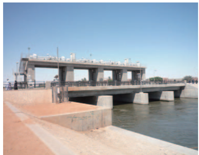
A rehabilitated and improved Sakoula Regulator (Egypt)
