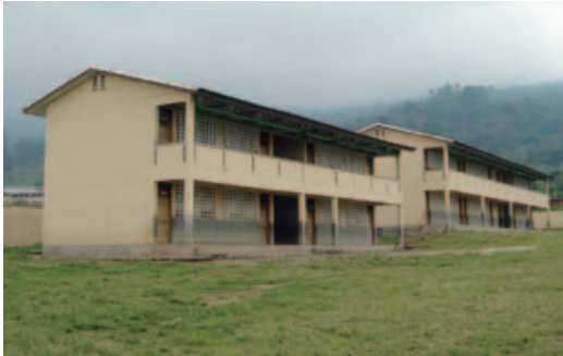
A school constructed by the project (Southwest Region)
