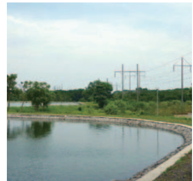
Stabilization pond at the wastewater treatment plant
