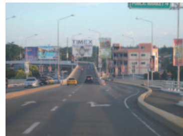
Ramp for left-turning vehicles on the Mactan Island side of the Second Mactan Bridge
