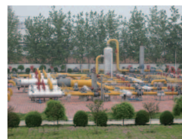
Gate stations receiving supplies of natural gas from the main pipeline (Zhumadian)
