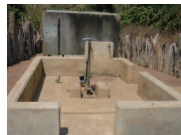
Foot-pumped deep wells with iron remover
