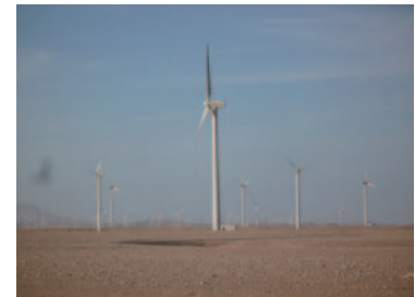
Wind power plant constructed in this project
