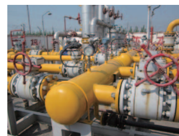
Pipeline, meters, and gauges used to make adjustments to gas pressure (Jiaozuo)
