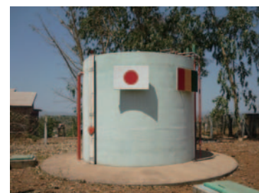
Water tank of piped water supply facility
