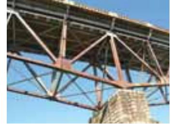
Rusted truss members of the Old Bridge
