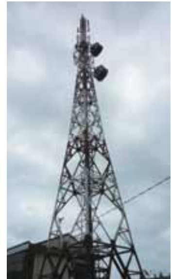
Microwave Transmission Tower
