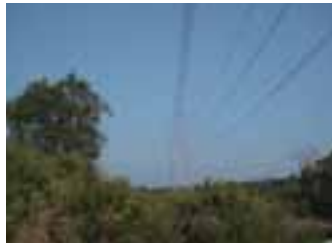
Transmission lines constructed under the project
