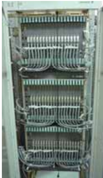
Digital Switching System
