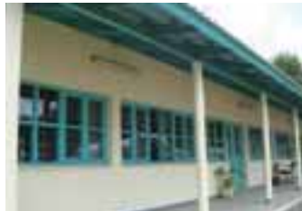
Constructed classroom (CFS* Massinga) * CFS : Training schools for health personnel; mainly at basic level
