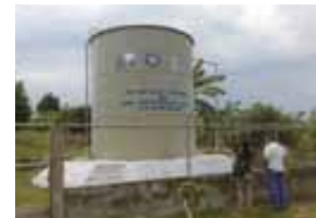
Water supply facility installed in LGU, South Davao Region
