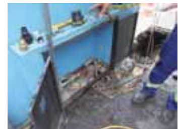
Replacement of water service pipes
