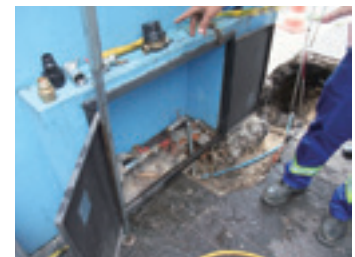
Replacement of water service pipes
