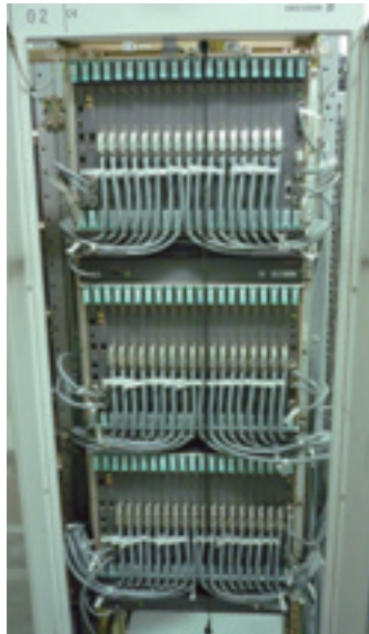
Digital Switching System
