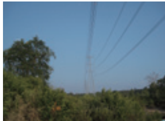
Transmission lines constructed under the project
