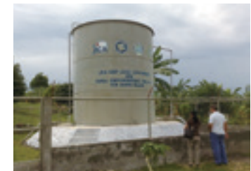
Water supply facility installed in LGU, South Davao Region
