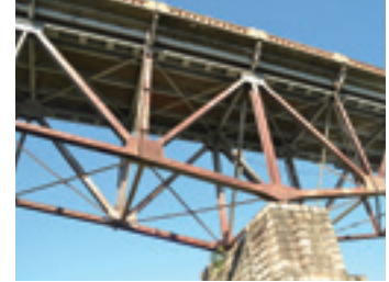
Rusted truss members of the Old Bridge
