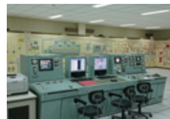
Engine Room Simulator Loaded on Board
