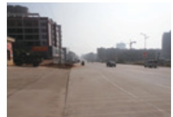
Zhushi-Chengbu Provincial Road
