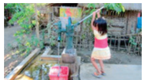
Deep hand pump well (level-1 water supply facilities) installed by Provincial Cities Water Supply Project (Phase 5) Calintaan, Occidental Mindoro (Taken from the ex-post evaluation report)
