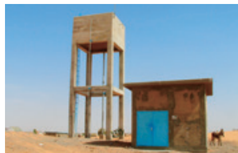
Boreholes with motor pumps and water supply facilities (elevated water tank and machinery house)
