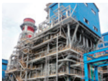
Heat Recovery Steam Generator
