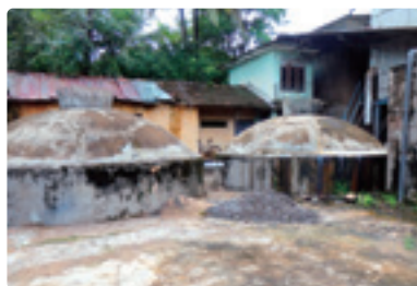
② Waste water treatment facility installed at a rice mill utilizing the sub-loan from this project
