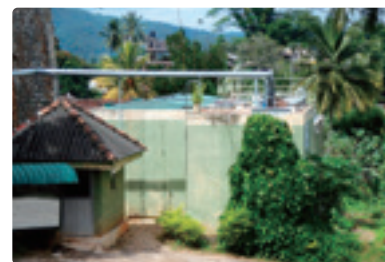
③ Waste water treatment facility installed at a hotel utilizing the sub-loan from this project
