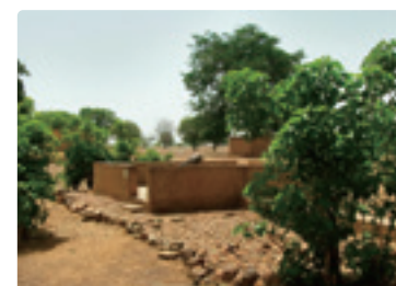
Gravel around the well, and hedge to avoid livestock animals (developed by the residents to avoid a mud puddle and scouring)
