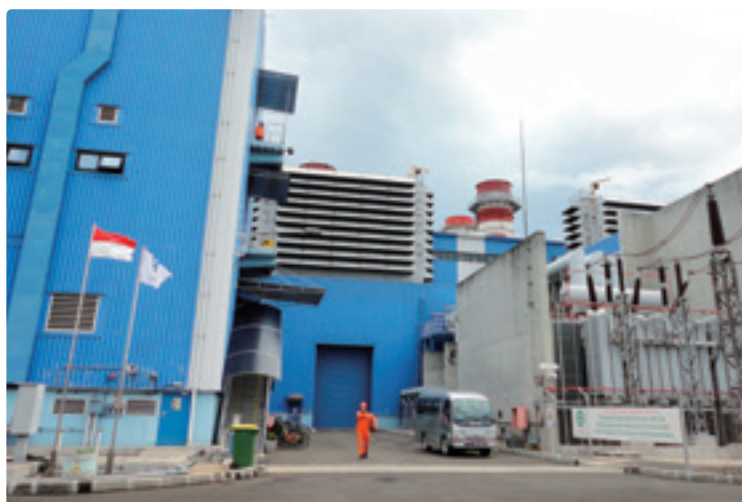
Tanjung Priok Gas Fired Power Plant
