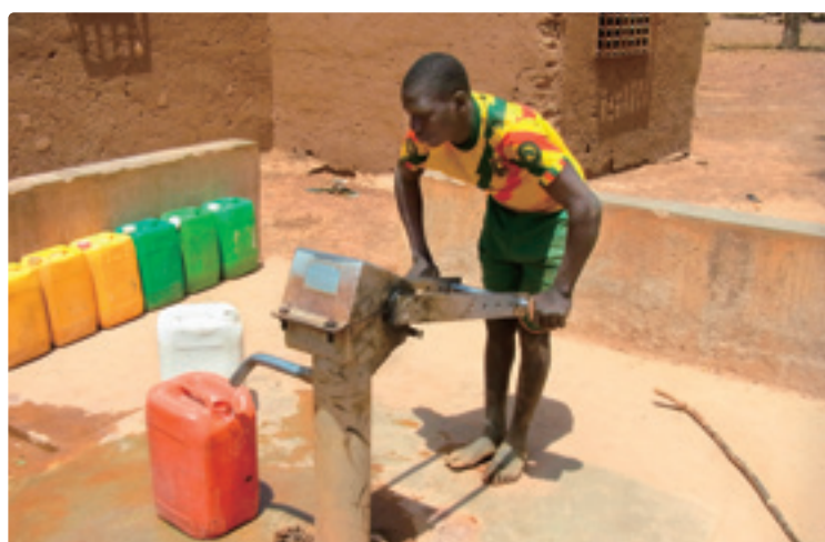
Deep well with hand-pump facility
