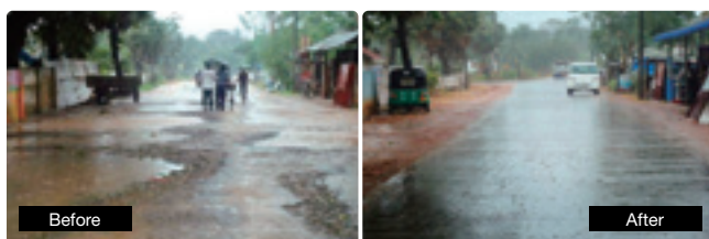
Before and after the road rehabilitation (photo provided by the implementing agency)
