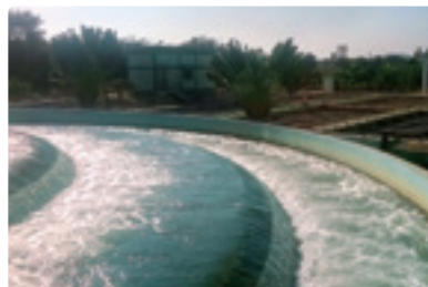
Water Treatment Facility (T.K. Halli)
