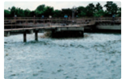
Sewerage Treatment Plant (Nagasandra)
