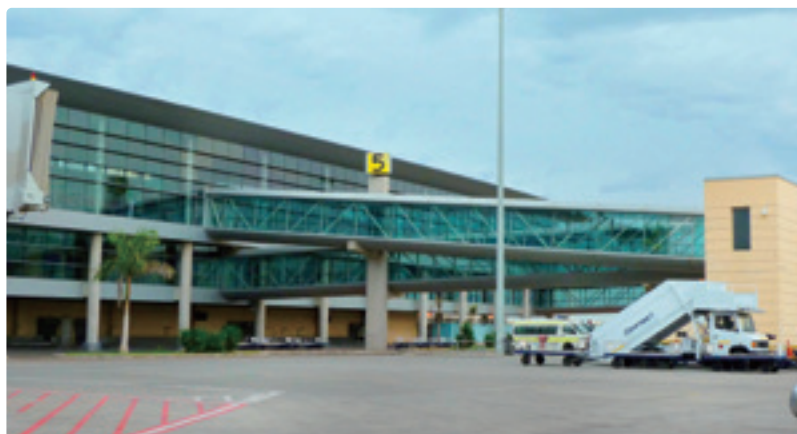
Passenger terminal constructed by the project
