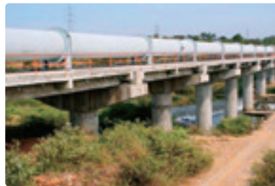
Water Transmission Line to Bangalore City
