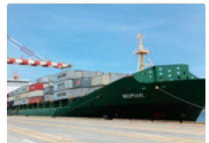
Container terminal constructed by Batangas Port Development Project
