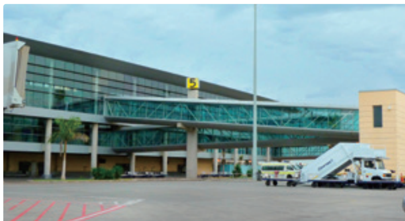
Passenger terminal constructed by the project
