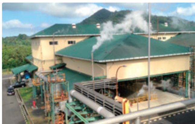
Lahendong Geothermal Power Plant
