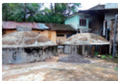
② Waste water treatment facility installed at a rice mill utilizing the sub-loan from this project
