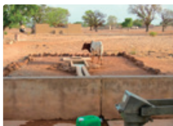
Livestock watering hole (spilled water from the pump flows to the hole through the drainage)
