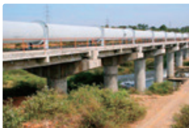
Water Transmission Line to Bangalore City
