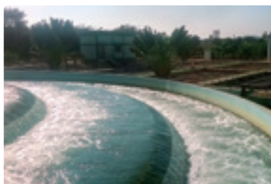
Water Treatment Facility (T.K. Halli)
