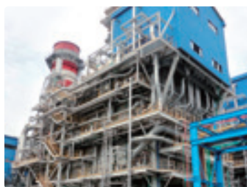
Heat Recovery Steam Generator
