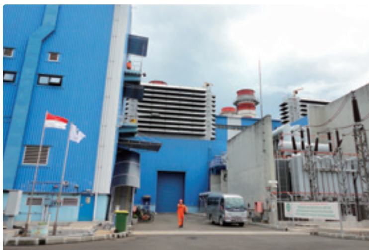
Tanjung Priok Gas Fired Power Plant
