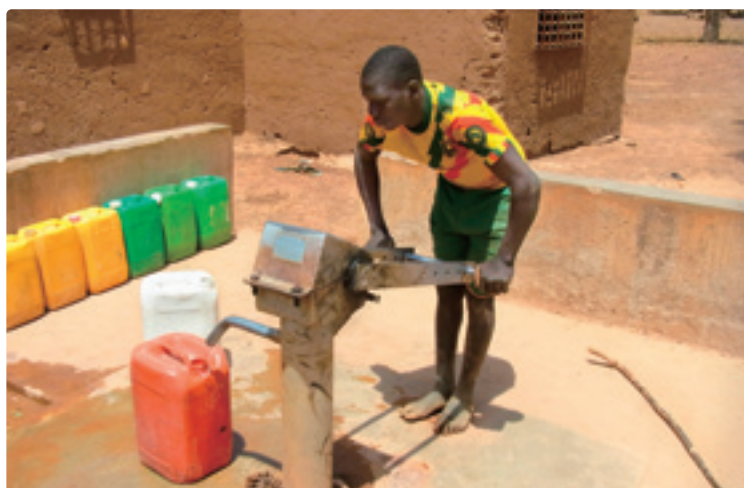
Deep well with hand-pump facility
