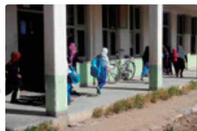
A school for girls constructed in Parwan Province in the Project for Construction of Basic Education Facilities in Afghanistan (Grant Aid)
