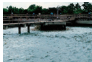
Sewerage Treatment Plant (Nagasandra)
