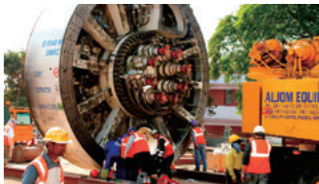
Assembling of a tunnel boring machine
