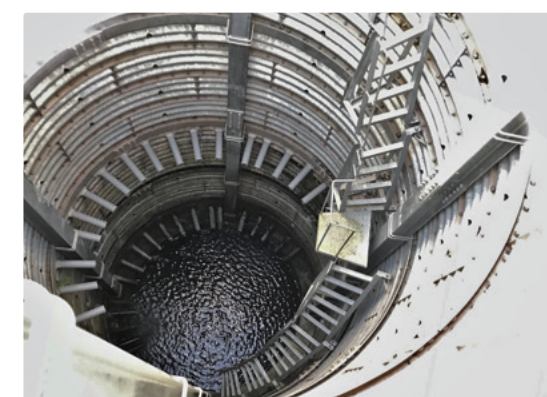
Catchment well and its interior in El Berrinche (water collection boring works deployed in a fan-like fashion can be observed)
