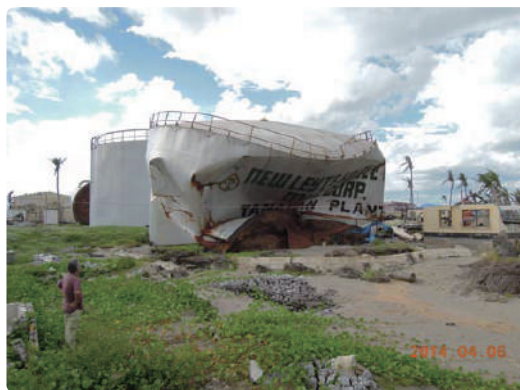
A coconut oil tank rolled over by typhoon, testifying its terrific force
