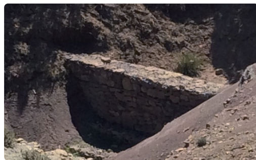
Check dams constructed to suppress the outflow speed of surface soil
