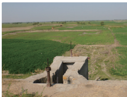
Water intake facility of a dam
