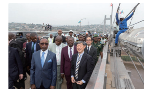
JICA President Kitaoka visited the Matadi Bridge in July 2019. Photo taken by Shinichi Kuno
