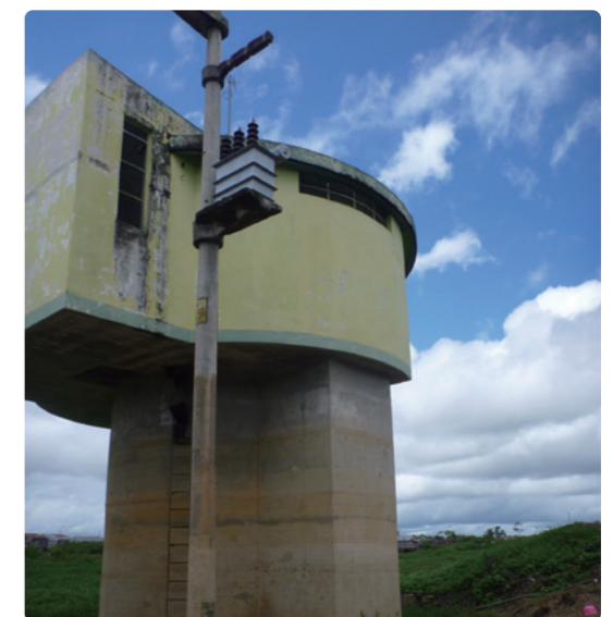
Pumping station constructed by the Project
