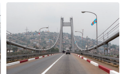
Main cables with the dry-air injection system installed. The city of Matadi located to the front. Photo taken by Shinichi Kuno
