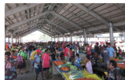
Internal view of the market building
