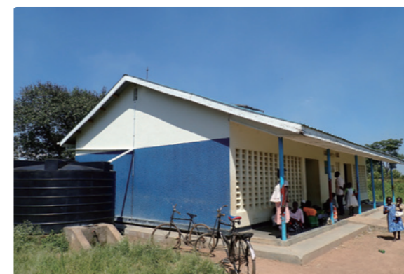
An outpatient ward improved by the project (Padel District)
