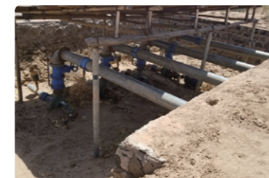
Irrigation facility constructed in Somali Region (Output 2)
