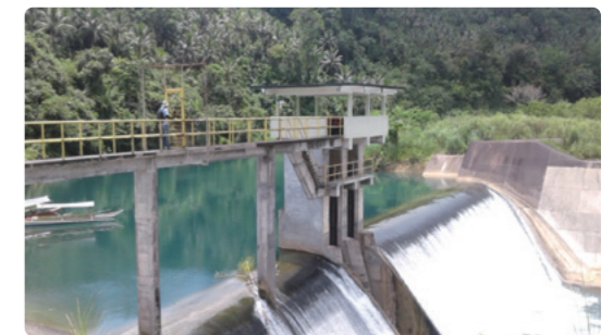
The completed Catubig Dam
