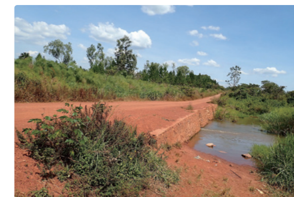
An access road and river crossings and road-drainage culverts improved by the project (Omoro District)
