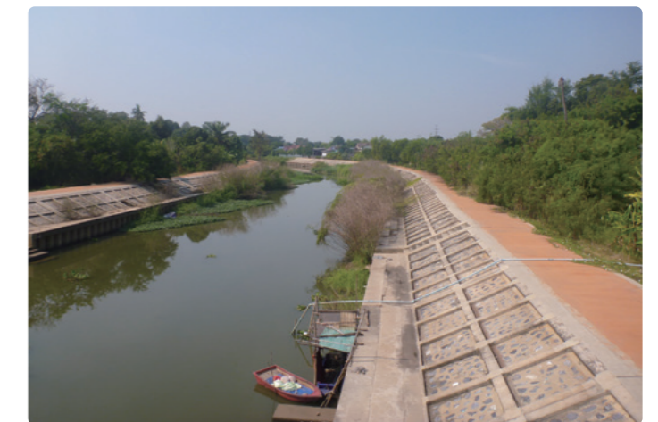
Banks of Hantra canal improved by the Flood Prevention Project of East Side of the Pasak River in Ayutthaya in Thailand
