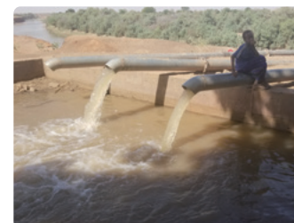
Irrigation facility constructed in Somali Region
