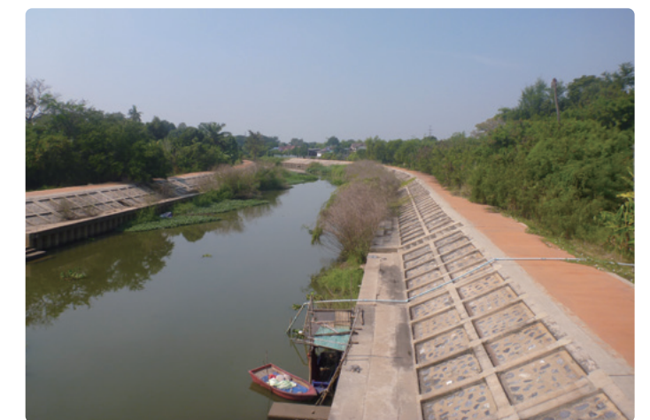
Banks of Hantra canal improved by the Flood Prevention Project of East Side of the Pasak River in Ayutthaya in Thailand
