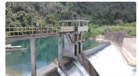
The completed Catubig Dam
