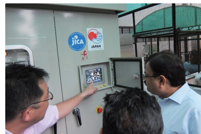
A survey conducted by the overseas office (Research Partnership for the Application of Low Carbon Technology for Sustainable Development in India)
