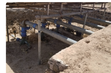
Irrigation facility constructed in Somali Region (Output 2)
