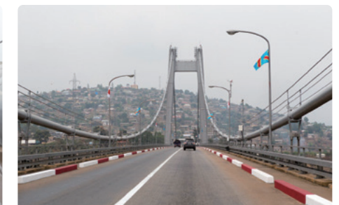
Main cables with the dry-air injection system installed. The city of Matadi located to the front. Photo taken by Shinichi Kuno
