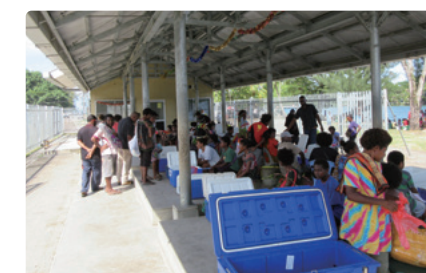
View of the fresh fish retail building
