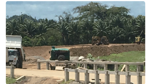
Main irrigation canal under construction in the Bulao Service Area
