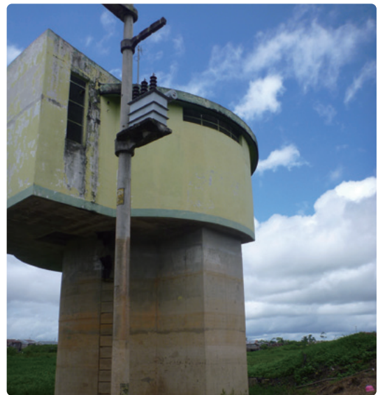
Pumping station constructed by the Project
