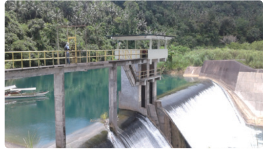
The completed Catubig Dam
