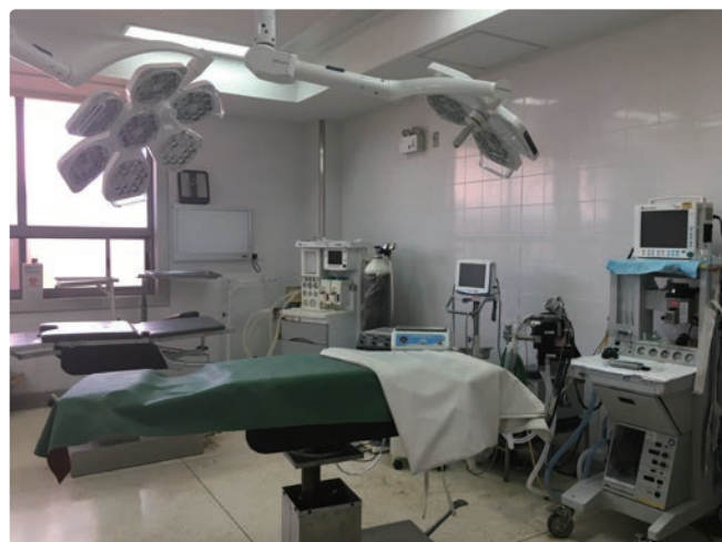
Constructed OT (Hoima RRH)
