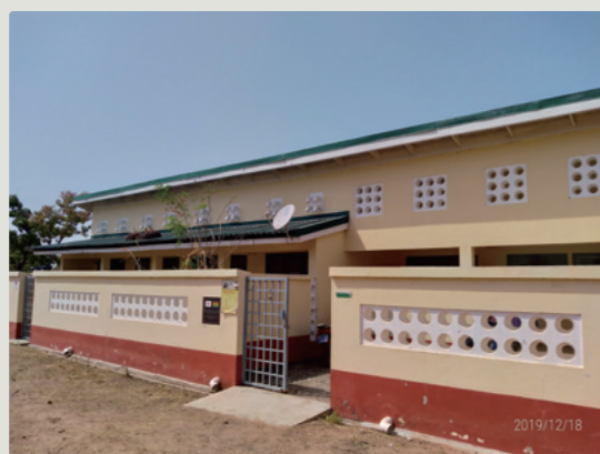
A CHPS Compound at the community where maternal and neonatal health services are provided
