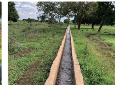
Canal developed by the project
