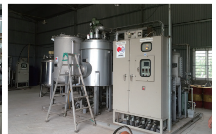
Analytical equipment provided by the SATREPS project at VNU
