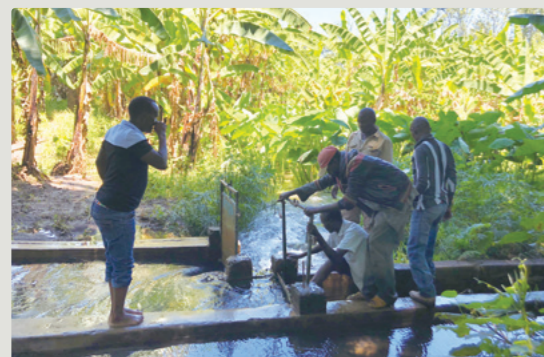
An intake weir constructed by the project and irrigation water users association members
