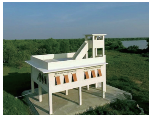
A cyclone shelter provided by the project
