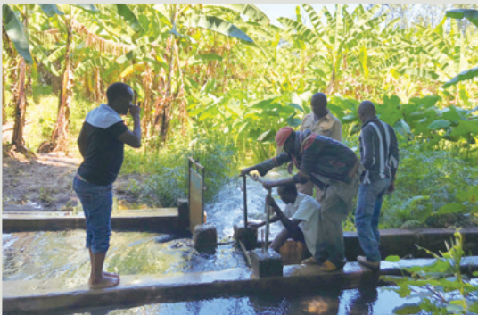
An intake weir constructed by the project and irrigation water users association members
