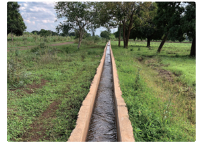
Canal developed by the project
