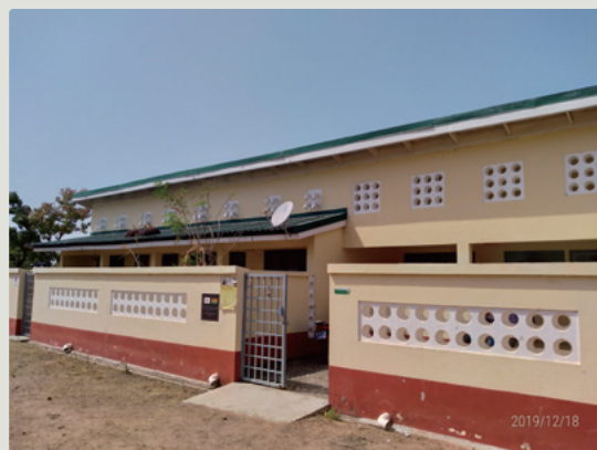
A CHPS Compound at the community where maternal and neonatal health services are provided
