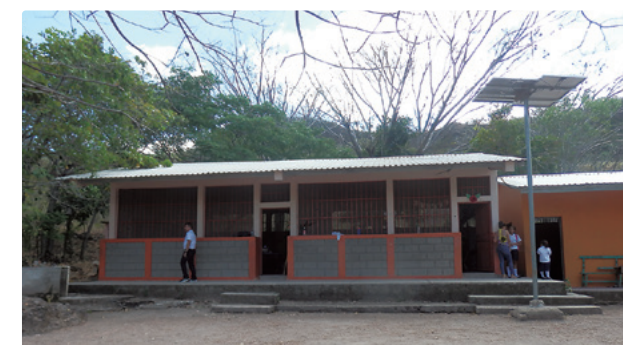
Classrooms built in accordance with the community development plan (Municipio de San Antonio del Norte)
