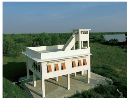
A cyclone shelter provided by the project
