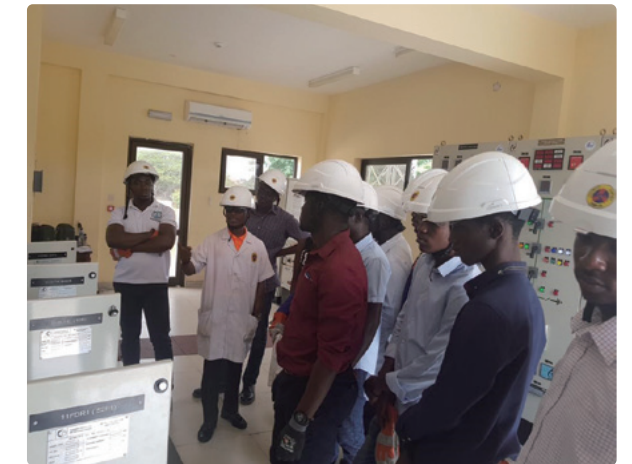
Training course for graduate engineers on multi skilling ("The Project on Electrical Engineers Training for African Countries (EETA)" in Ghana)
