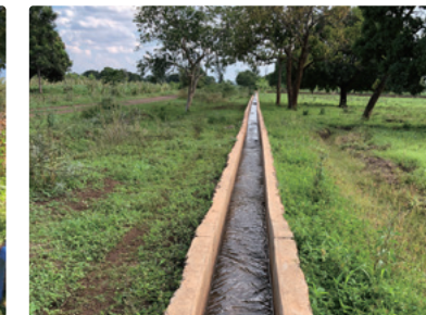
Canal developed by the project
