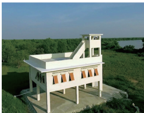
A cyclone shelter provided by the project
