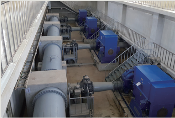
Transmission and distribution pumps installed by the project at the Nyaunghnapin First Phase Water Treatment Plant
