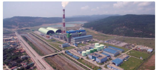
A panoramic view of the Power Plant (Nghi Son Thermal Power Plant Construction Project in Viet Nam)
