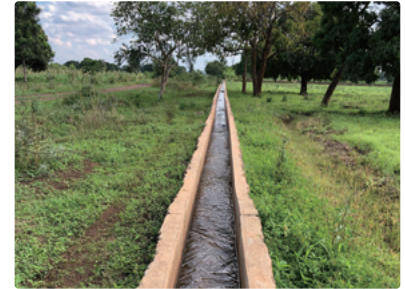
Canal developed by the project
