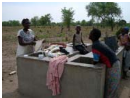
Photo4 Washing Slab in Delampuli
