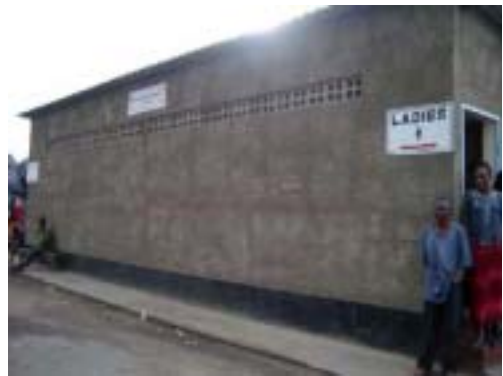
Photo5 Public Toilet by GCEP, George
