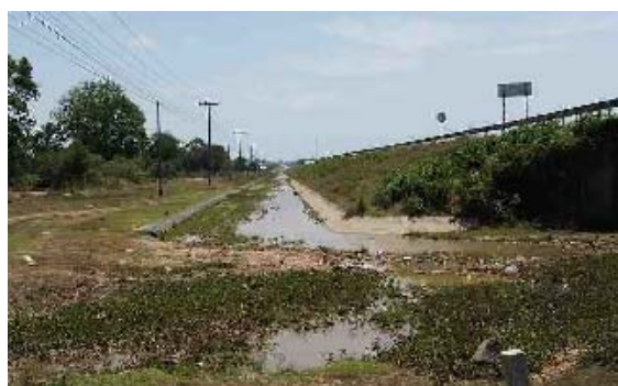
Photo 4: Drainage on north side of NR9
