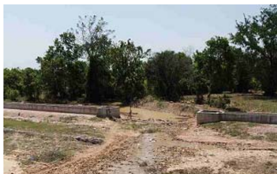
Photo 5: The situation on the side of Houay Koa Bridge
