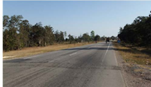
Photo 1: Start Point of Section 1
