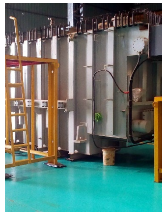
Transformer under repair
