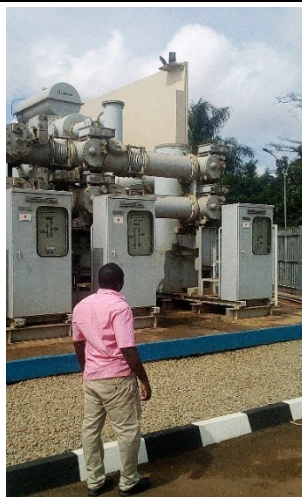
Outdoor 132 kV gas insulated switchgears
