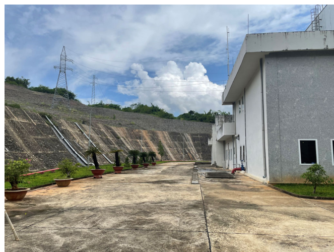
Exterior of the Thac Mo Hydropower Station
