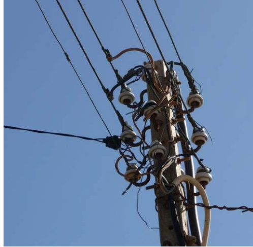
Figure 2.2 Deteriorative PMT and LV line
