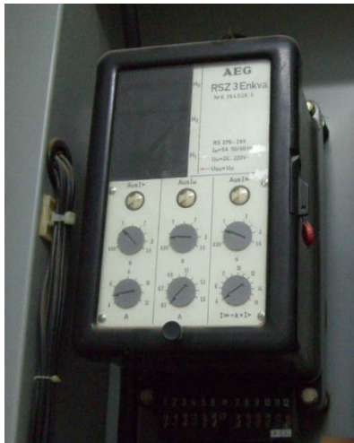
Figure 2.5 Old Protection Relay and Circuit Breaker
