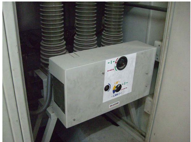
Figure 2.5 Old Protection Relay and Circuit Breaker
