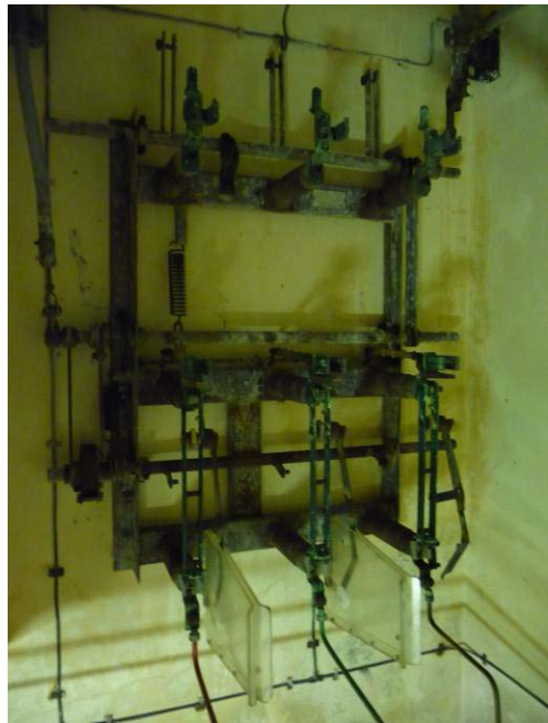
Figure 2.3 Deteriorative secondary substation and bus-bar
