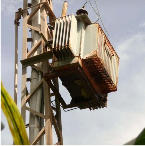
Figure 2.2 Deteriorative PMT and LV line
